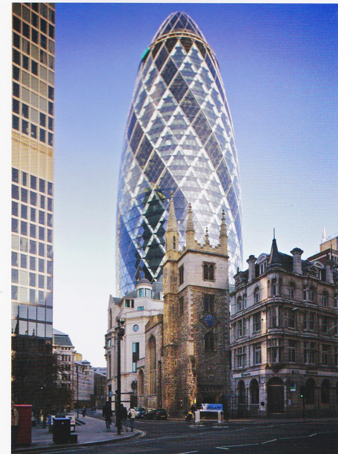
Fig. 15. Foster + Partners, Swiss Re Headquarters in London, 1997–2004. Photograph by Aurelien Guichard, Creative Commons.
